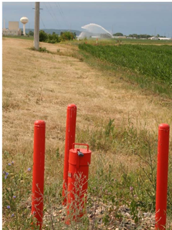
Groundwater monitoring wells north of the Village.
