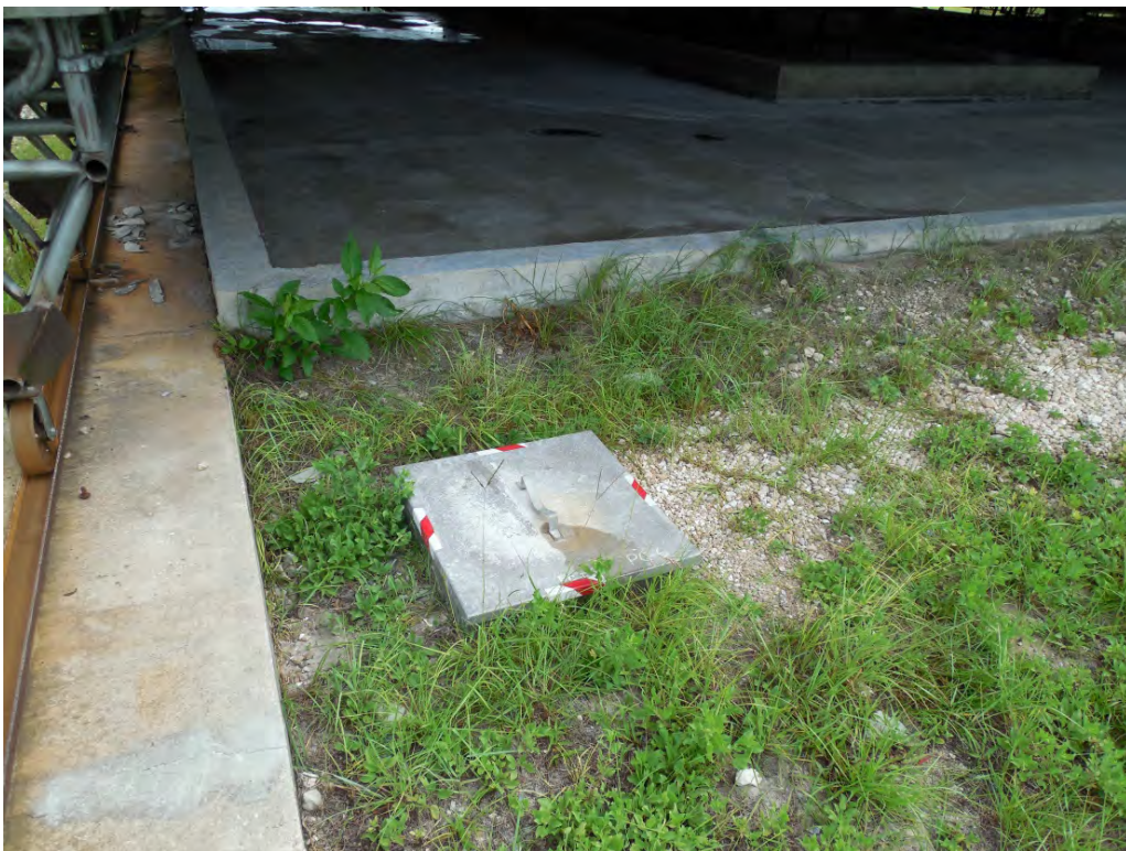
Photo 20: Similar view of the proximity of monitoring well to the OBU structure.
