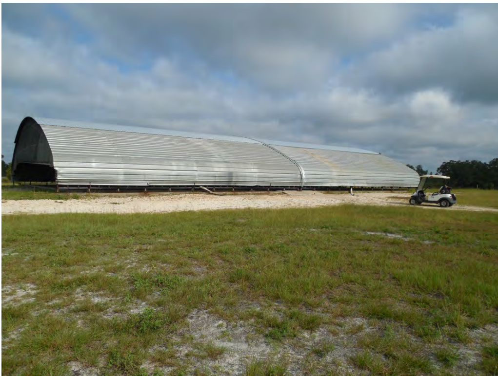
Photo 10: View of the OBU from the east.
