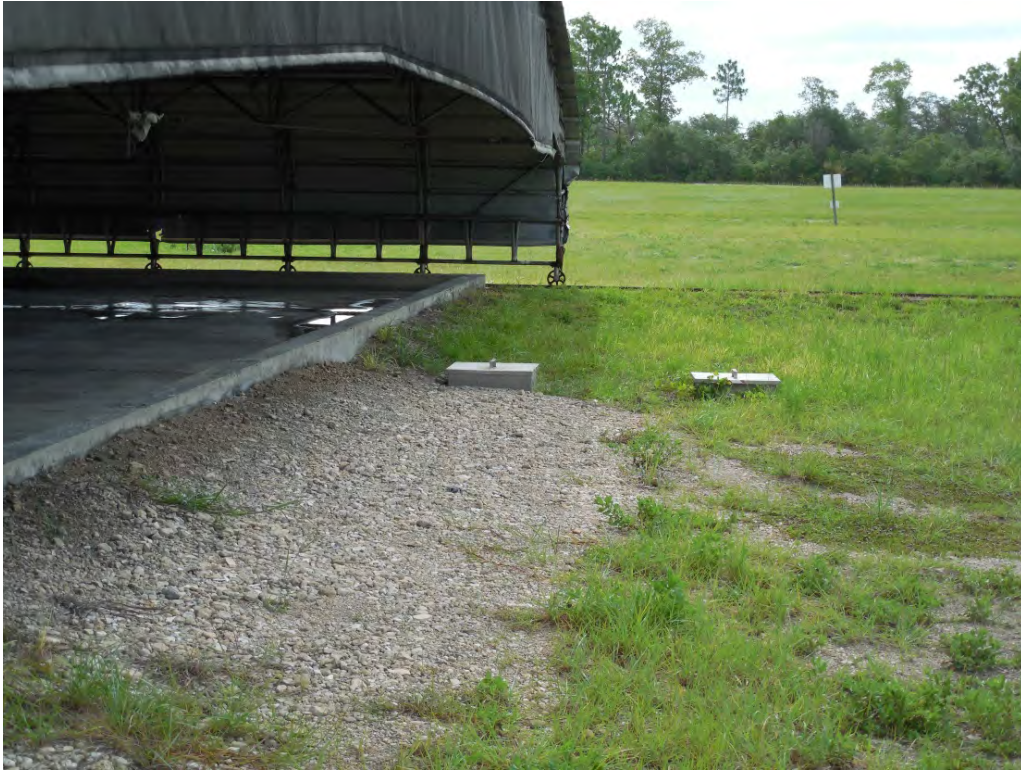
Photo 15: Northern portion of the OBU, depicting previous land subsidence repair efforts.
