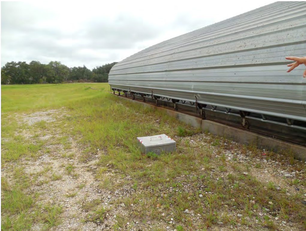
Photo 19: Proximity of monitoring well to the OBU structure.
