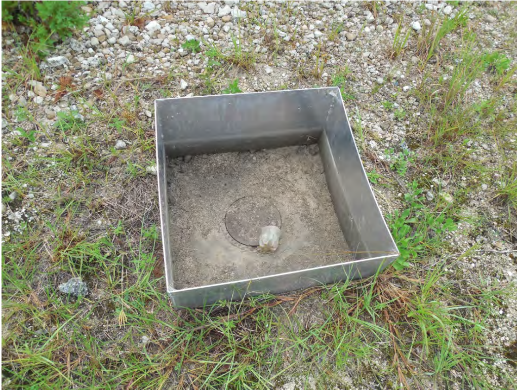
Photo 17: Damaged monitoring well proposed for replacement.
