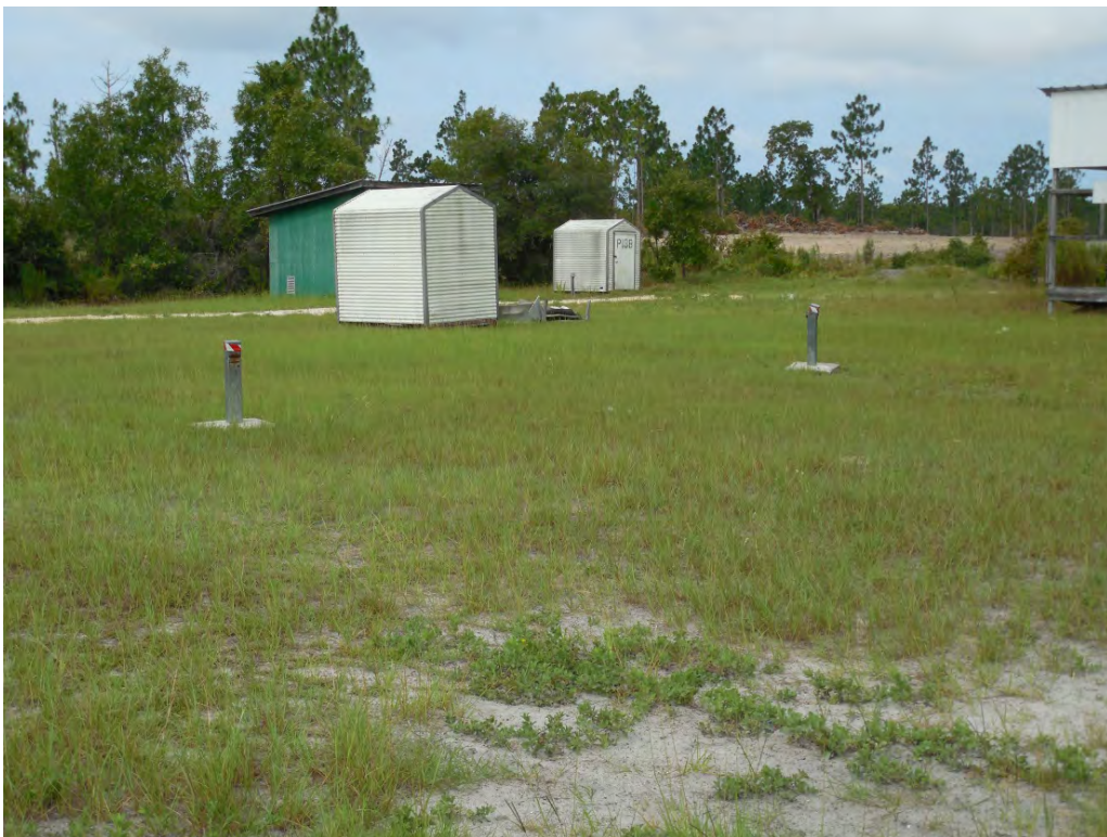
Photo 12: Portable storage buildings and monitoring wells south of the OBU.
