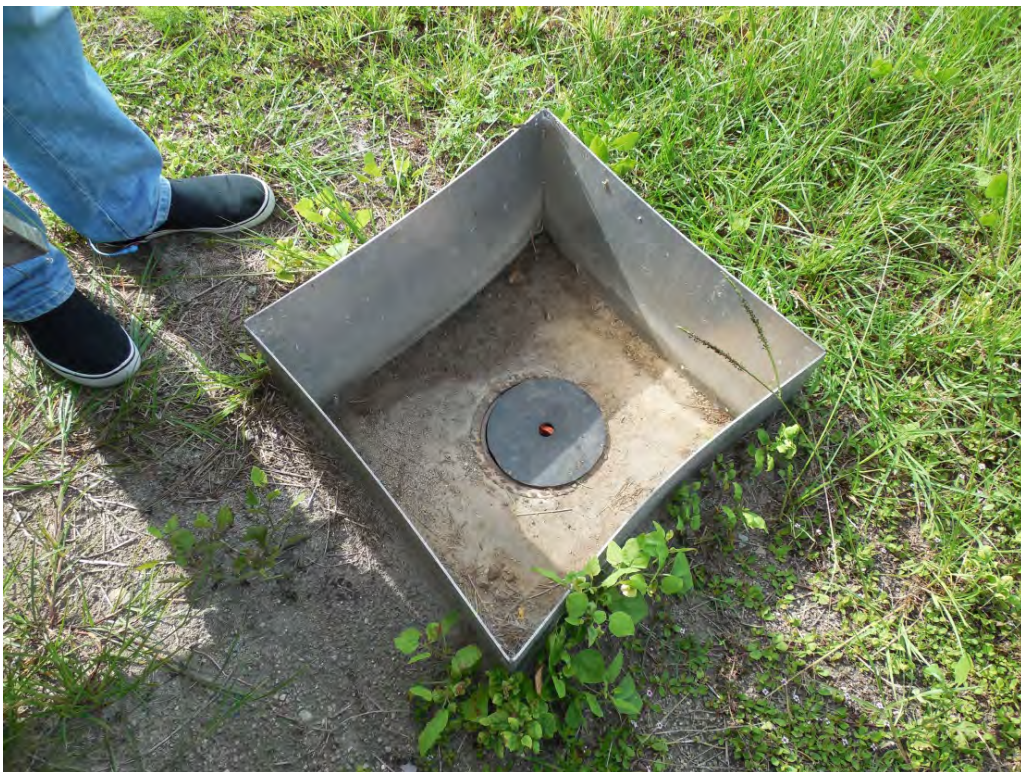
Photo 18: Similar view of damaged monitoring well proposed for replacement.
