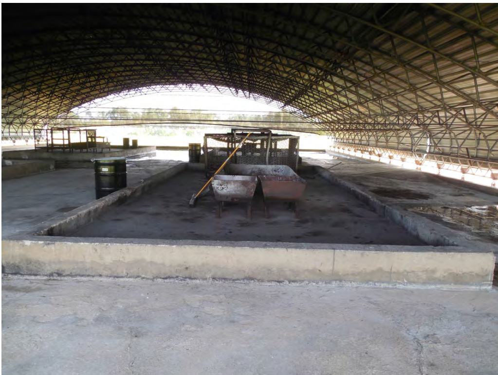
Photo 2: Interior portion of the OBU, facing south.
