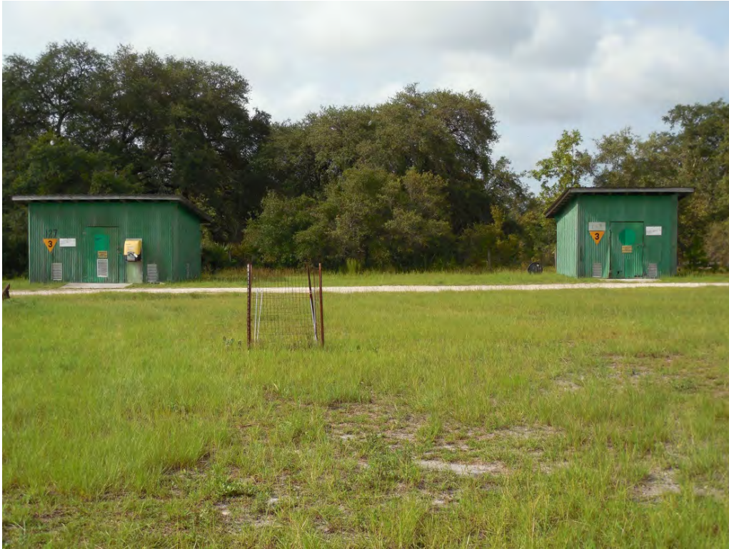
Photo 11: Waste storage buildings south of the OBU.
