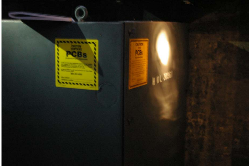
Bldg 8 A Transformer unreadable HOL ID number
