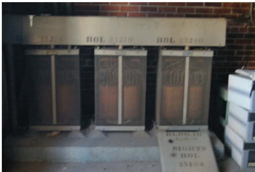
Bldg 7 A unknown capacitor bank PCB concentration
