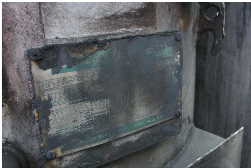
Bldg 200 PCB Transformer L495603PMLB
