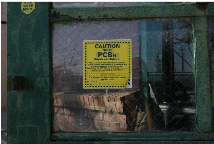
Bldg 20 A PCB Large Mark
