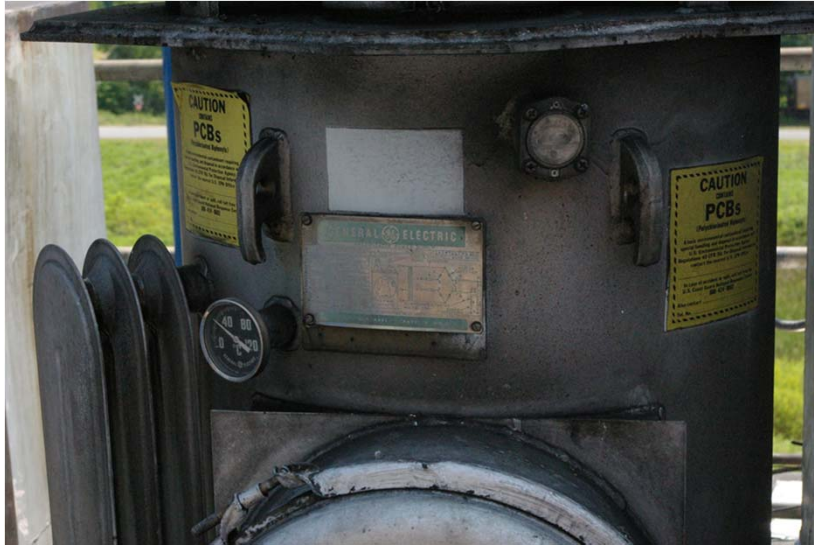
Bldg 200 PCB Transformer L495599PMLB
