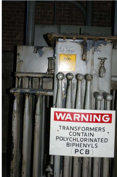
Bldg 8 A Transformer HOL 35811
