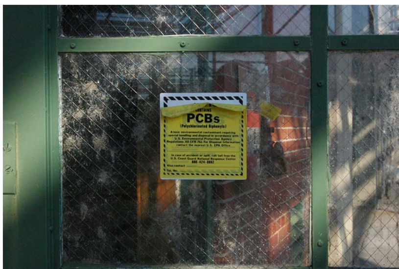
Bldg 7 A Large Mark
