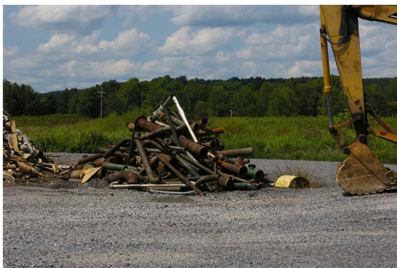
Burn Pile possible lead based painted pipe
