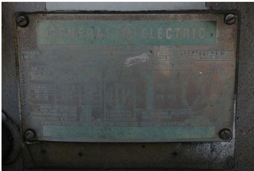
Bldg 200 PCB Transformer L495599PMLB
