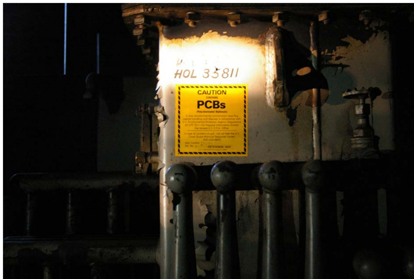
Bldg 8 A Transformer HOL 35811
