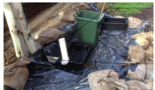
Site preparation, outside of discharge end of pipe
