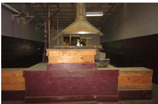
Equipment and building fixtures inside bay area
