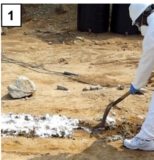
MuniRem® mixed into contaminated soil
