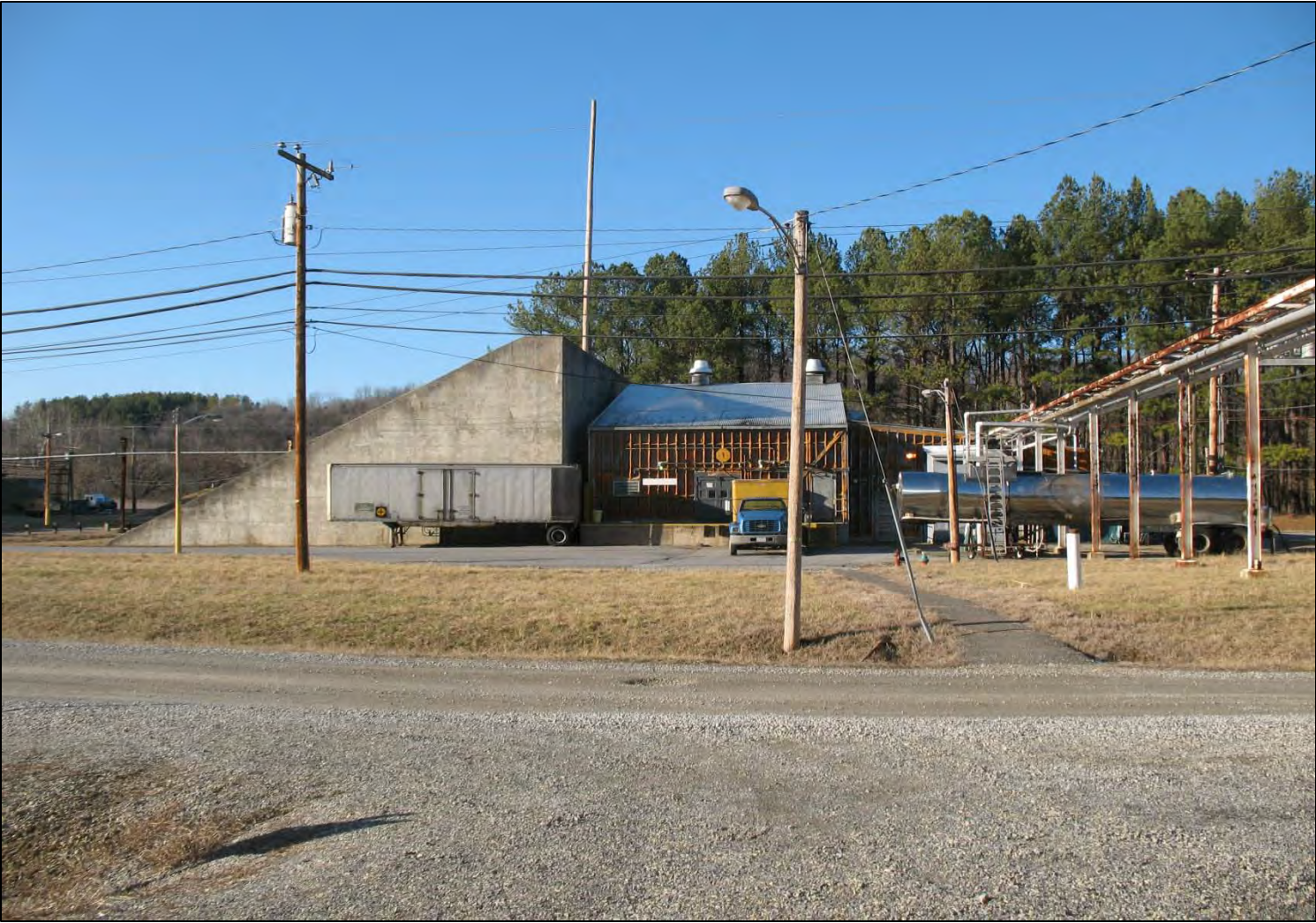
Figure 4. Pre-incinerator Grinder Bldg 442 (Process Code T04 – February 2012)
