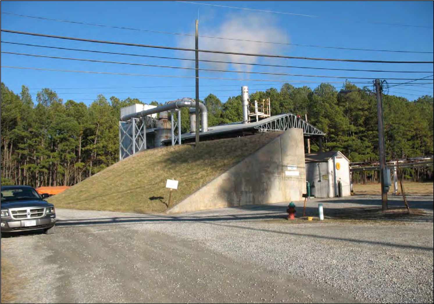
Figure 6. Incinerator 441 (Process Codes S02 and T03 – February 2012)
