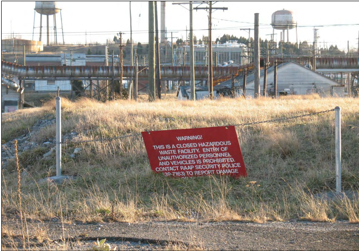
Figure 8. Hazardous Waste Management Unit 5 (Post Closure Care Permit – February 2012)
