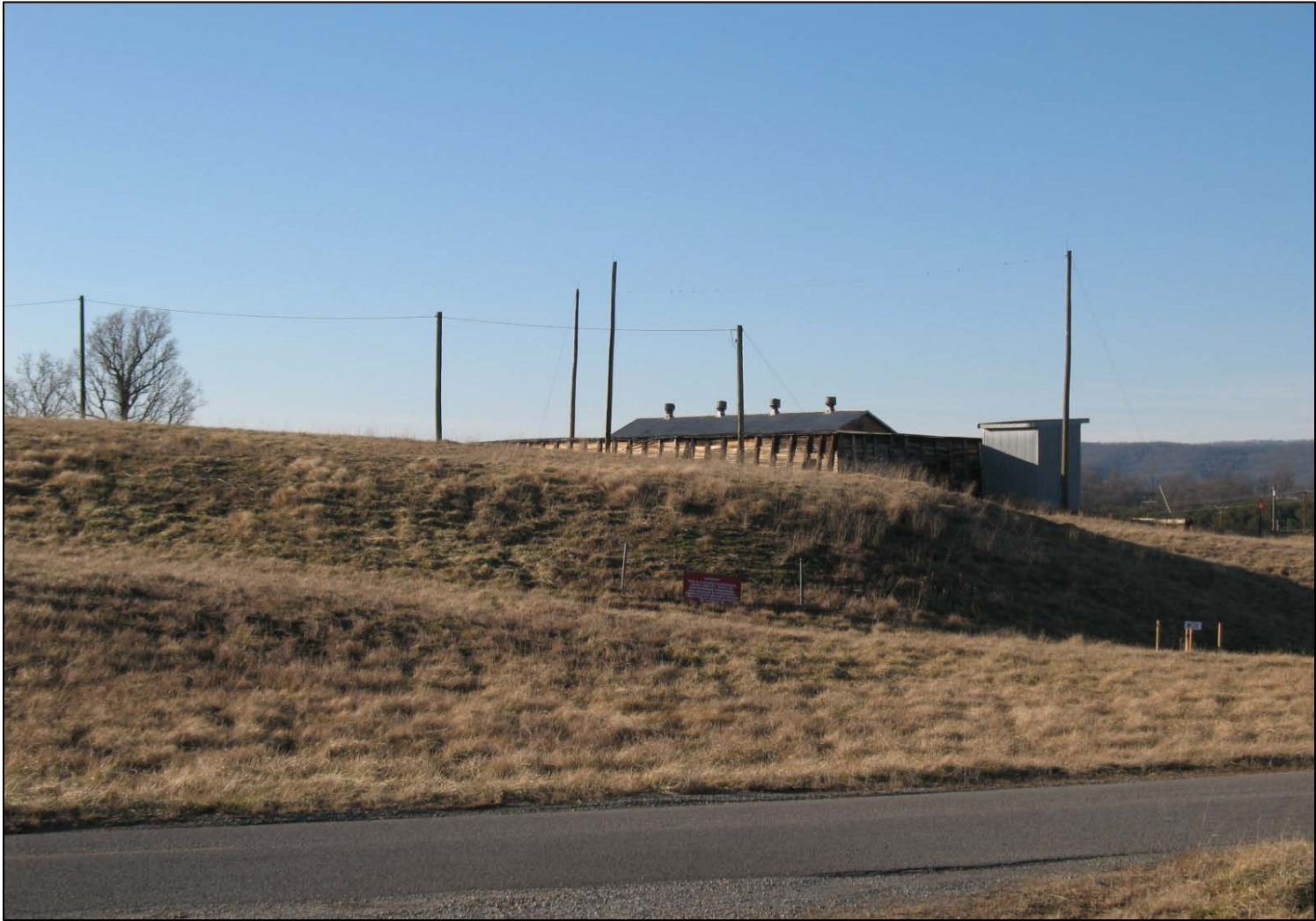
Figure 9. Hazardous Waste Management Unit 16 (Post Closure Care Permit – February 2012)
