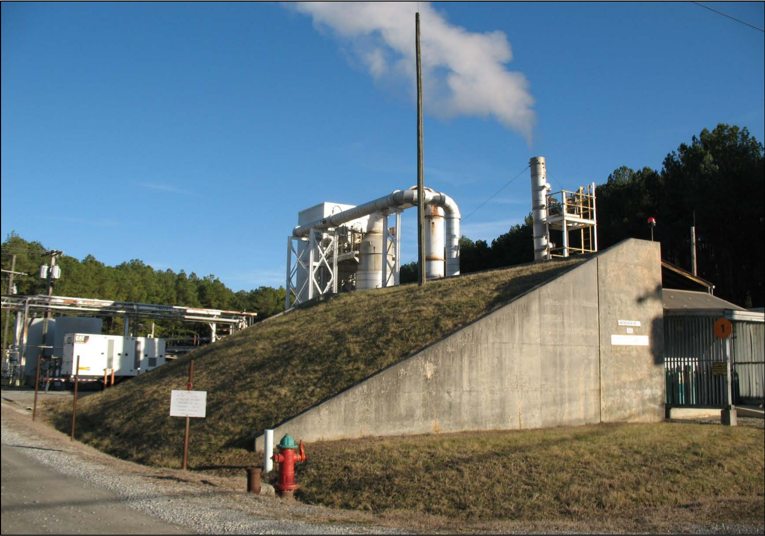
Figure 5. Incinerator 440 (Process Codes S02 and T03 – February 2012)
