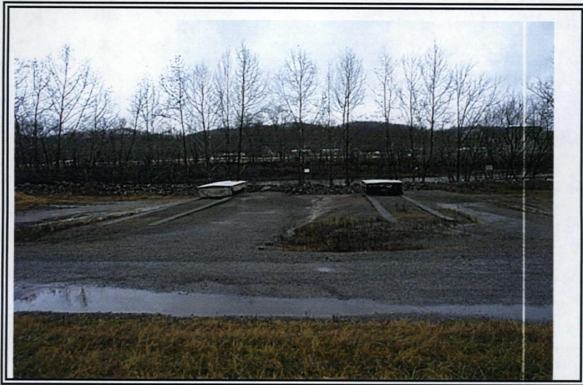
Photograph No. 2. View of the south of two pans comprising one pad.
