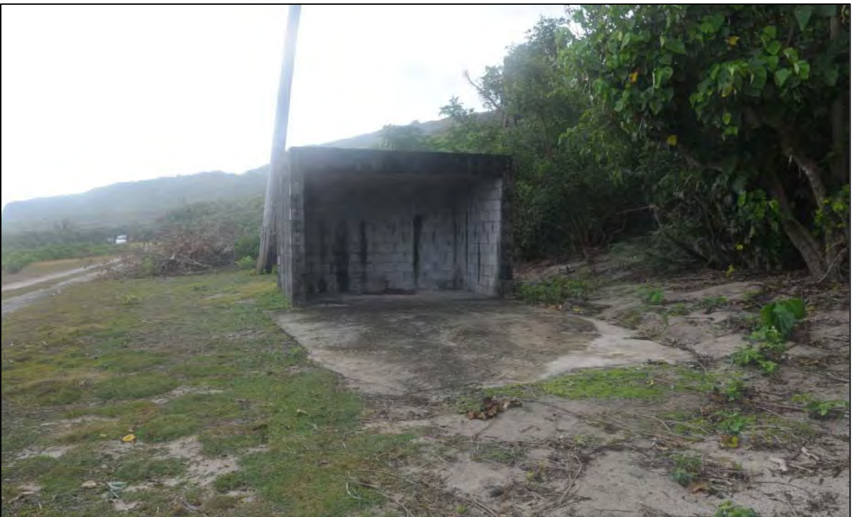
Photo 4. Cement/personnel bunker (looking east)
