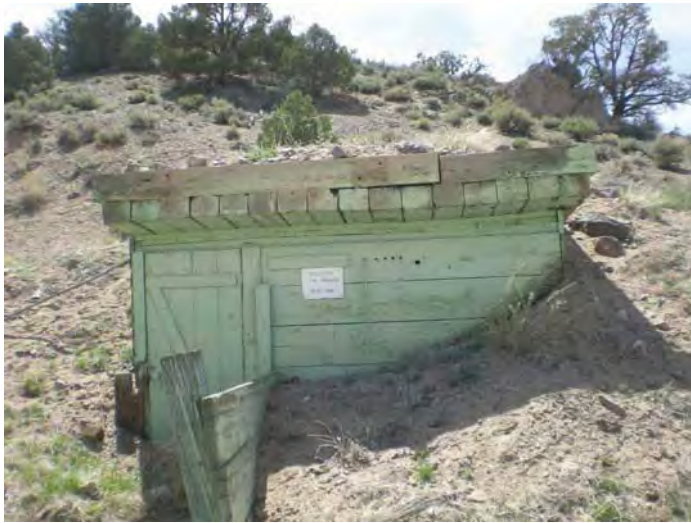
Storage Shed No Longer Used
