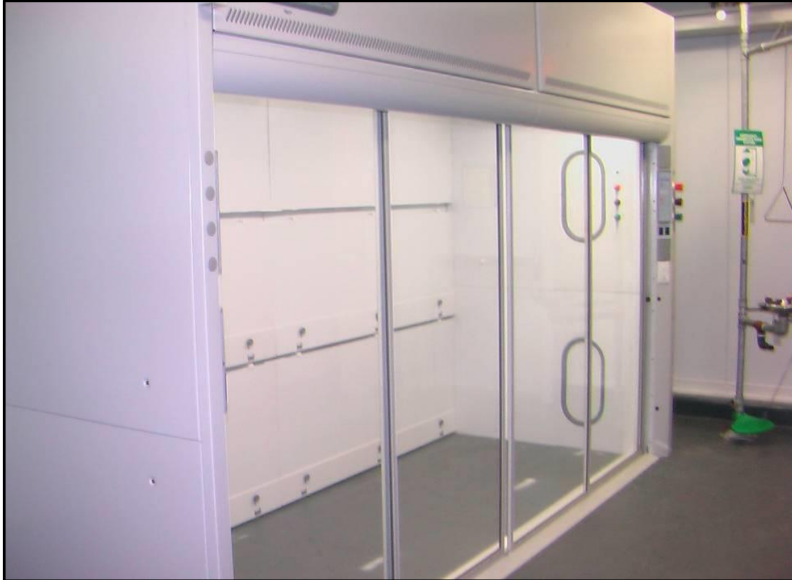
Figure 32. Walk-In Fume Hood
