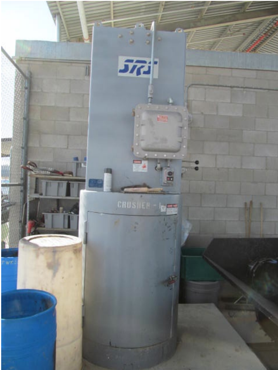
HWSTF Container Storage Area Process Code X02 (Block 7; Line 06)
