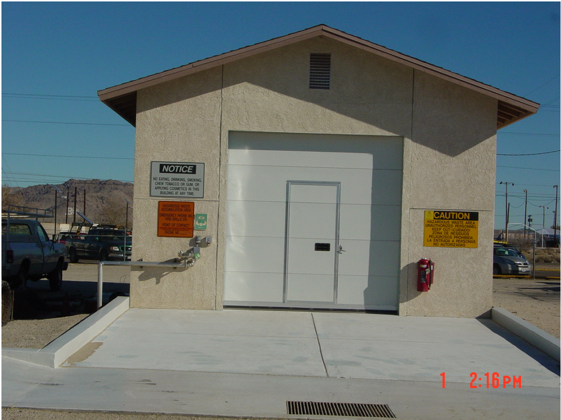
PCB Storage Building Process Code S01 (Block 7; Line 03)
