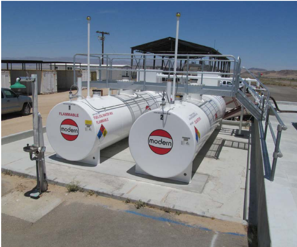
HWSTF Waste Oil Tanks Process Code S02 (Block 7; Line 02)
