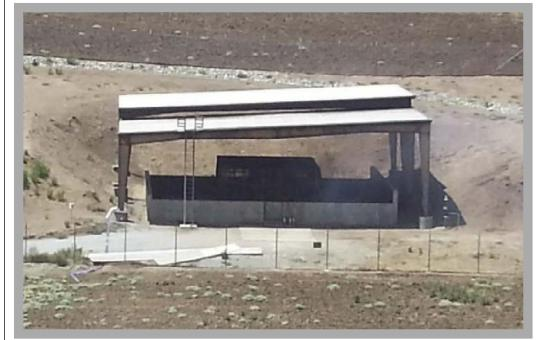
TSU-1 contains two 10-foot diameter, reinforced concrete pipes (burn tubes) which are enclosed in a reinforced, expanded metal mesh cage (22' W x 28' D x 10'10" H). The mesh cage is surrounded by concrete walls, installed in 2002, and on three sides by an earth bank and earth barricades over 15 feet high.
