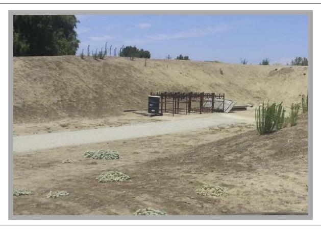
Explosive hazardous waste in solvent (EHWS) is burned in open horizontal, split steel troughs supported by steel racks in a double boiler arrangement. Contaminated solvents containing relatively more water or lower volatility are placed in the upper container. The fire is initiated remotely in the lower container. EHWS is not placed into the unit until just before burning is started. The treatment capacity is 300 gallons per day.
