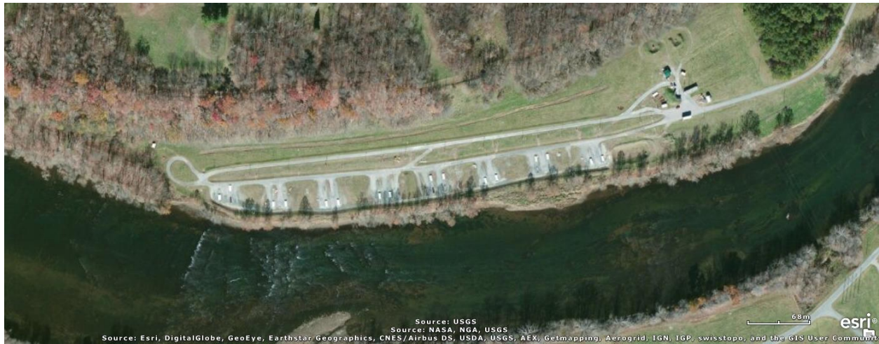
Figure 2-1. Overhead View of RFAAP Burn Pan Site.
