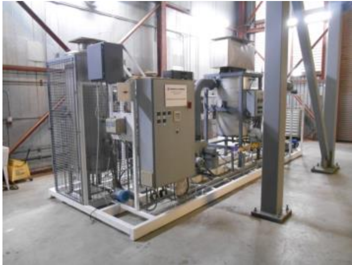
iSCWO System used for different chemical waste treatment tests
