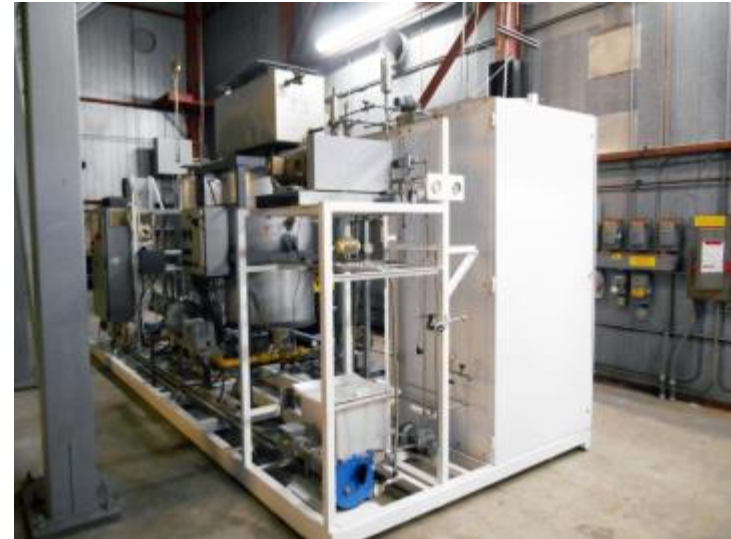
Dedicated iSCWO Test Facility
