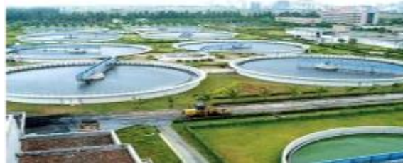
Sewage Concentrate destruction
