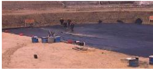
Ground water cleanup
