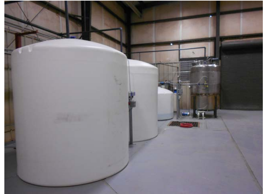
3 GPM iSCWO Tanks
