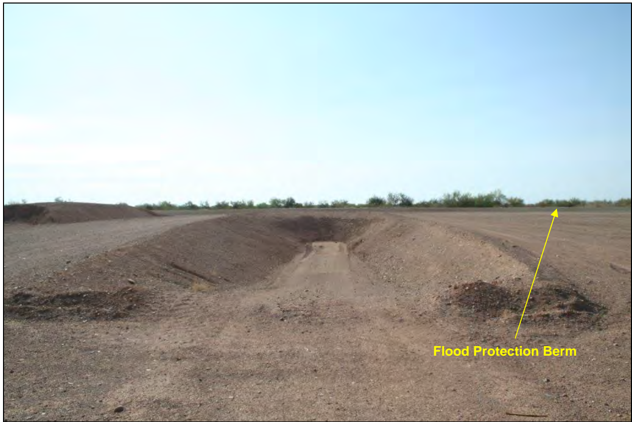
Photo 13 – Munitions Treatment Facility Detonation Pit #2 Trench (1 of 2) Facing Southeast and Southeast Inside Edge of Flood Protection Berm
