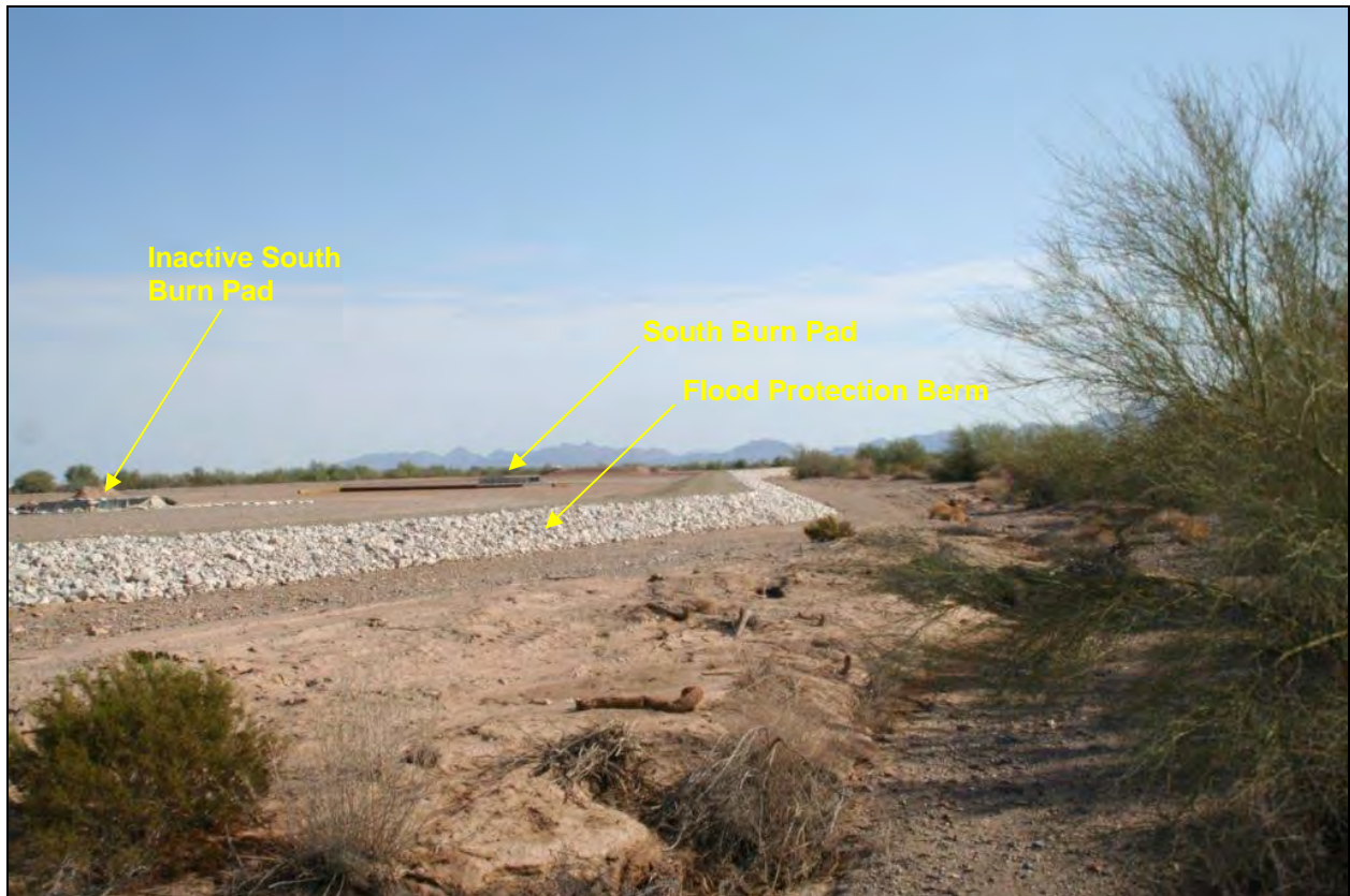
Photo 16 – Outside Southeast Edge of Munitions Treatment Facility Flood Protection Berm Facing Northwest to the South Burn Pad
