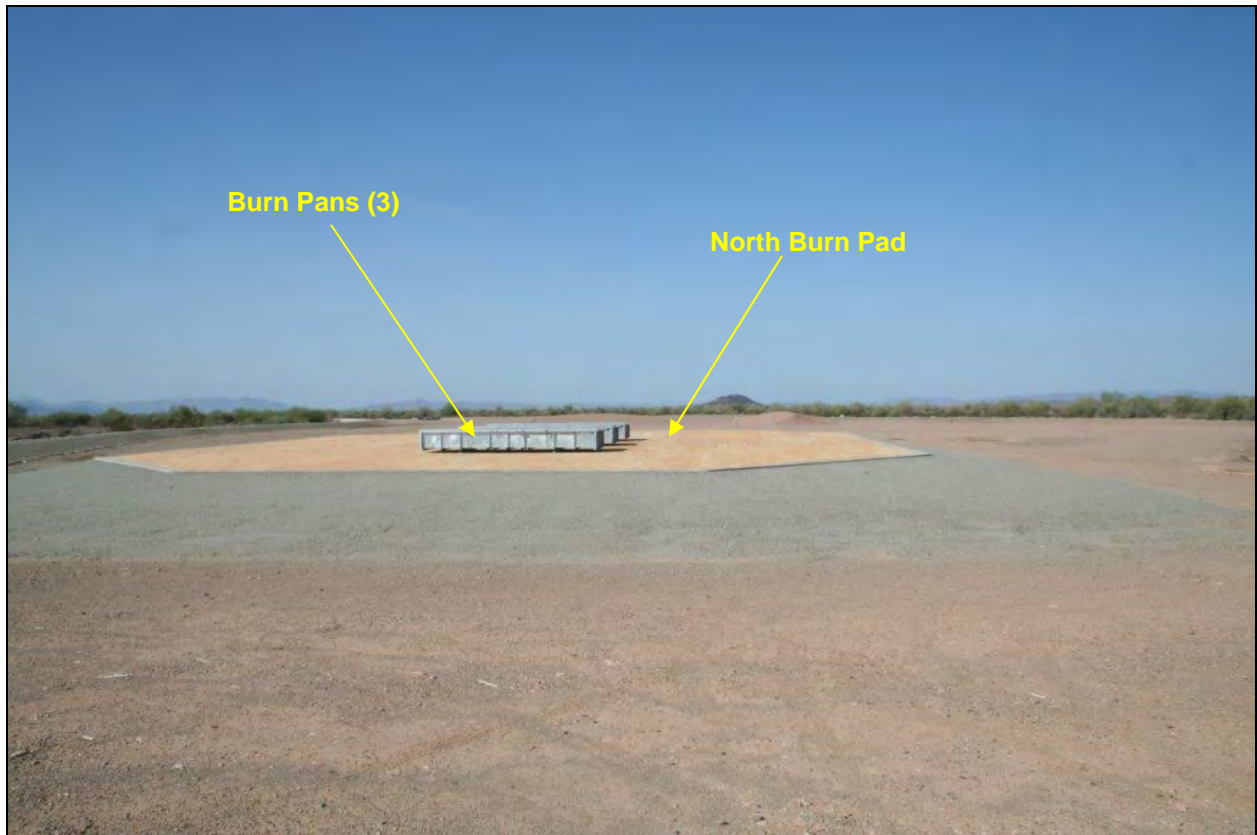
Photo 10 – Munitions Treatment Facility Facing Southwest Towards the North Burn Pad and Burn Pans (3)
