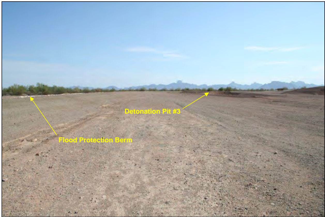
Photo 5 – Inside of Munitions Treatment Facility Flood Protection Berm Northeast of Entry and Detonation Pit #3
