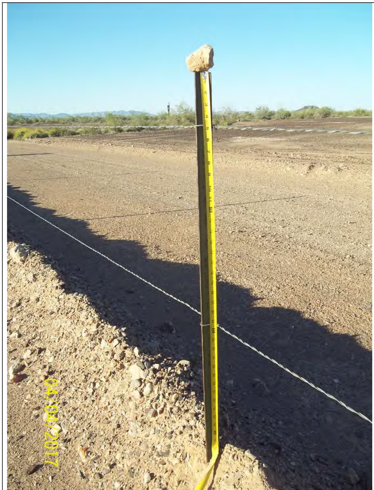
Photo 2 – Close-up of OB/OD MTF Perimeter Fencing Showing Wire Strands At Approximately 24-Inches Above Grade (24-Inch Mark on Ruler) and 43-inches (5-Inch Mark on Ruler)
