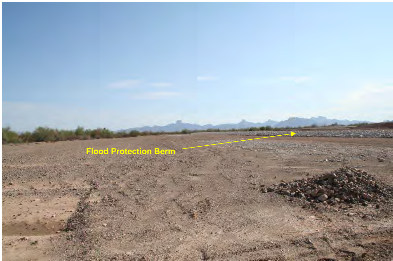
Photo 4 – Outside of Munitions Treatment Facility Flood Protection Berm Northeast of Entry
