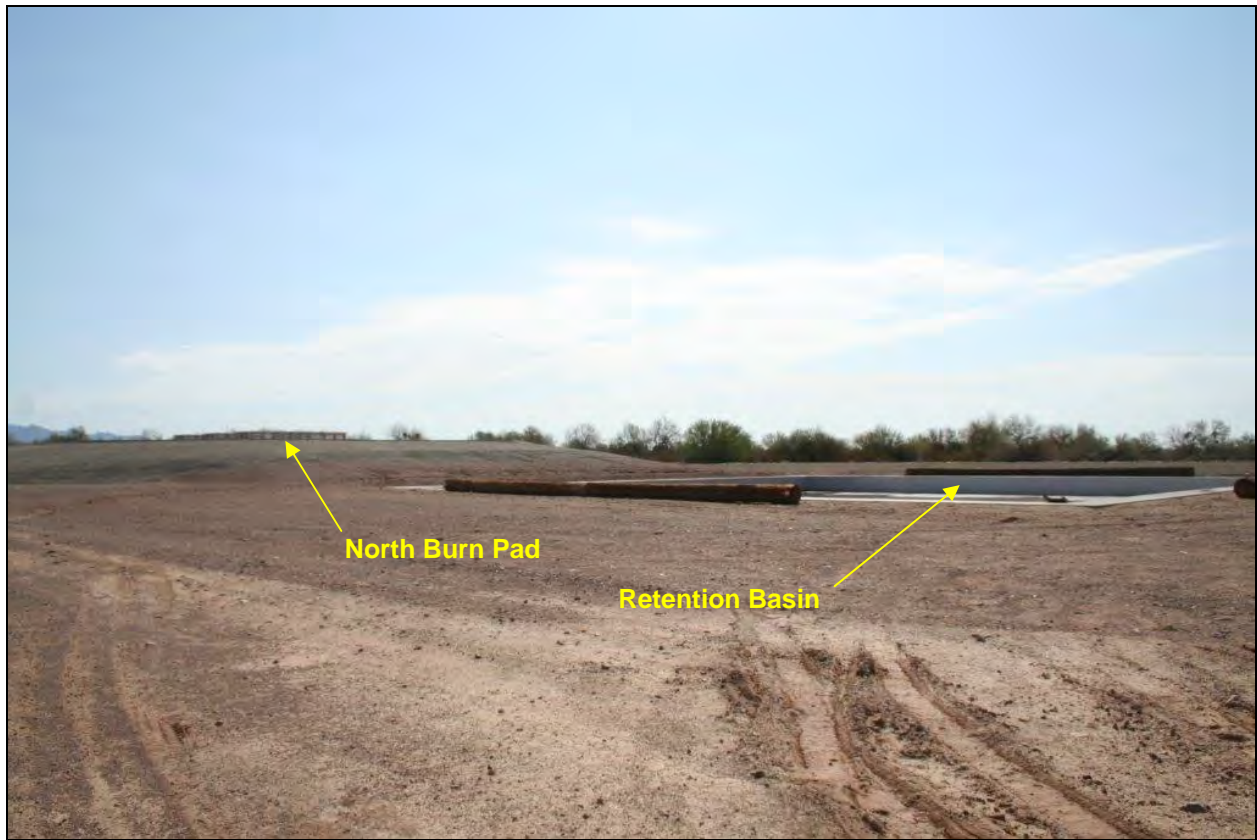
Photo 9 – Munitions Treatment Facility Facing Northeast Towards the North Burn Pad and Retention Basin
