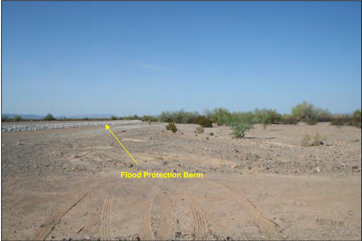
Photo 2 – Outside of Munitions Treatment Facility Flood Protection Berm Southwest of Entry
