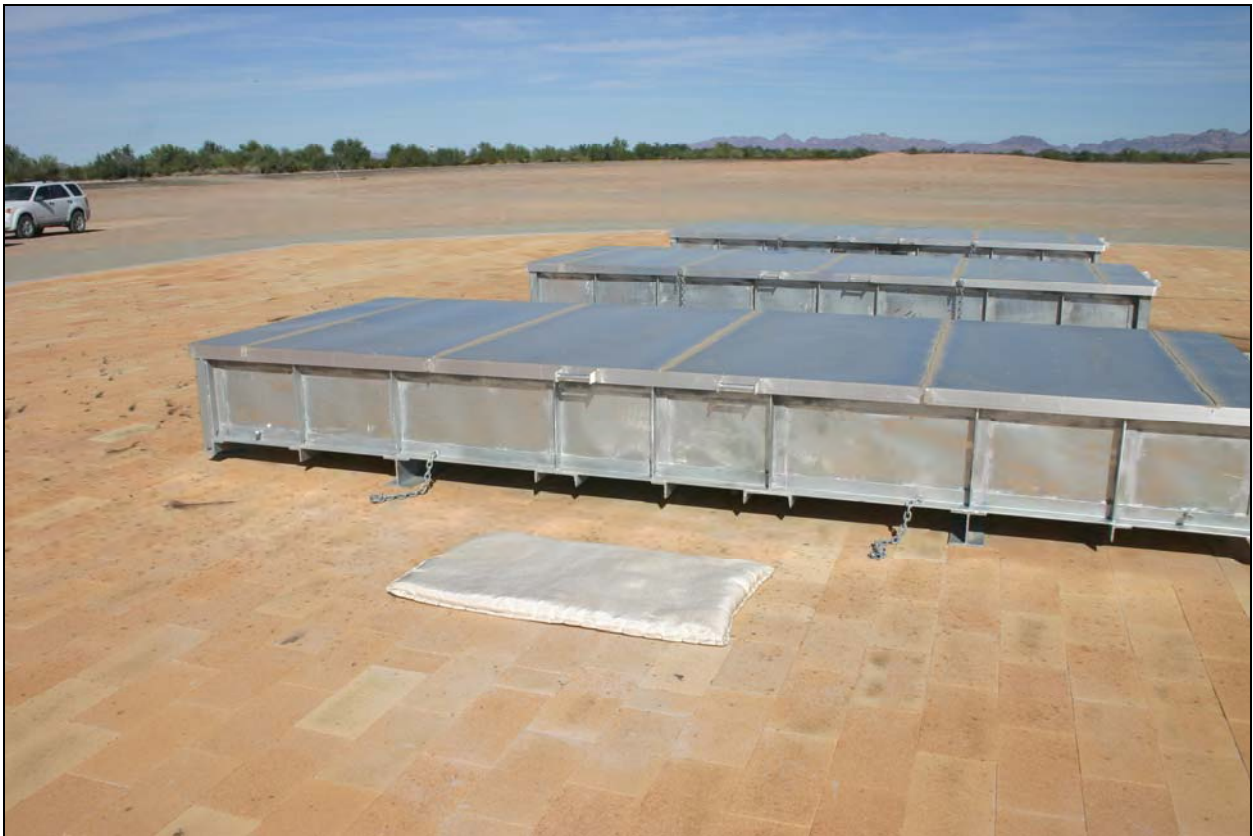
Photo 19 – Munitions Treatment Facility South Burn Pad and Burn Pans (3)
