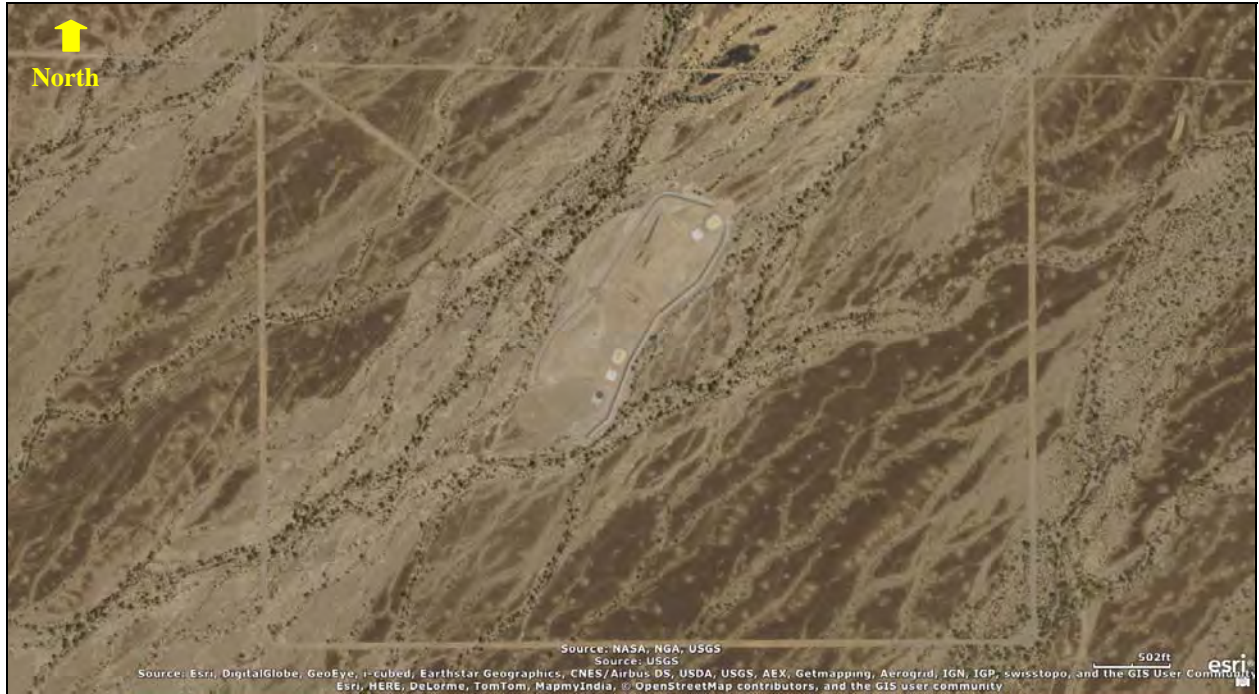
Aerial Image 1 – Munitions Treatment Facility Perimeter
