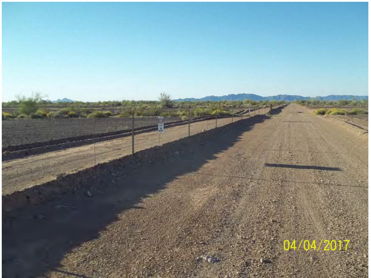
Photo 1 – OB/OD OB/OD Munitions Treatment Facility Perimeter Wire Fencing With 48-Inch High Metal Posts (measured from road surface to top of post).
