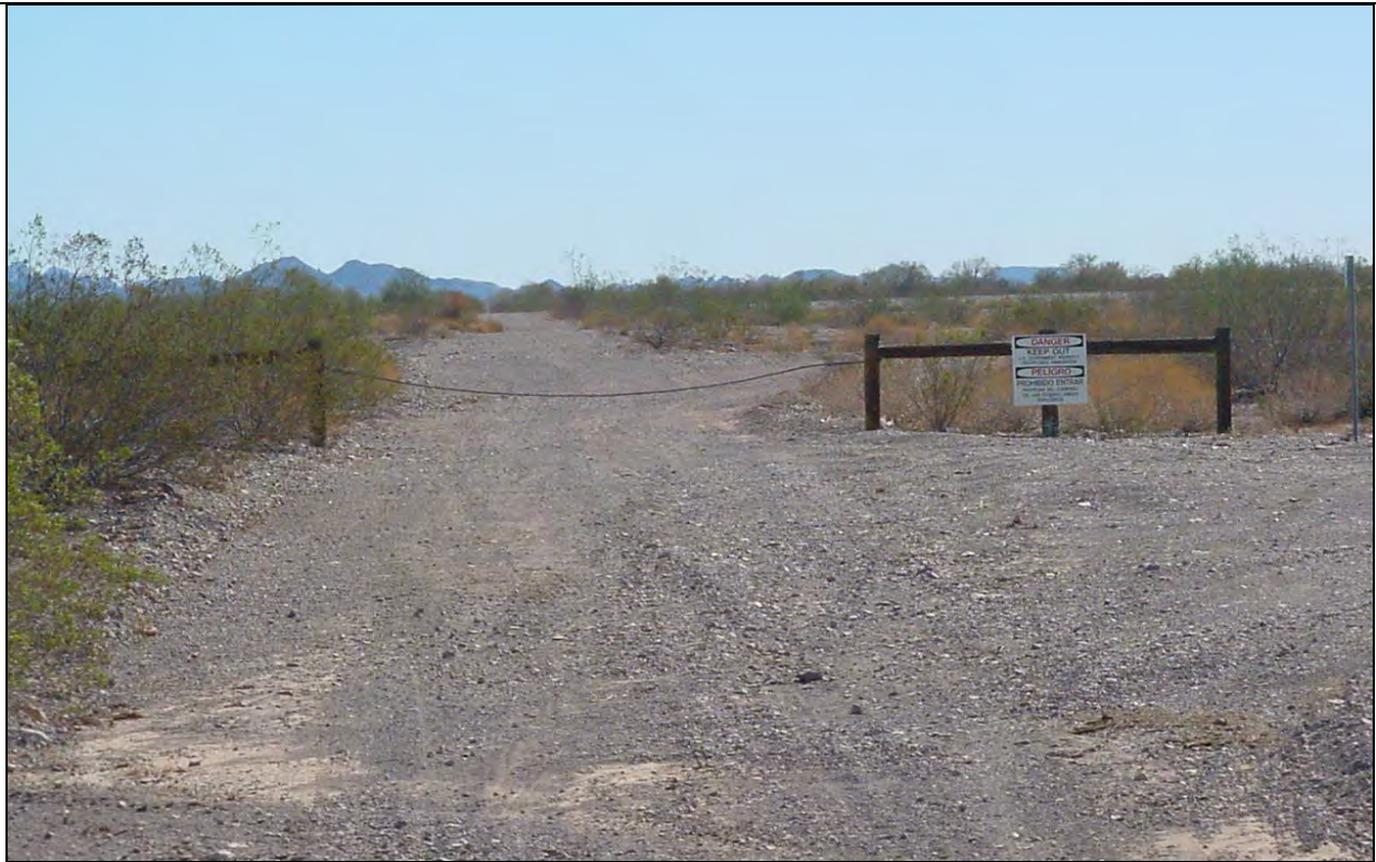
Photo 4 – Fence and West Gate Entrance to the OB/OD Munitions Treatment Facility
