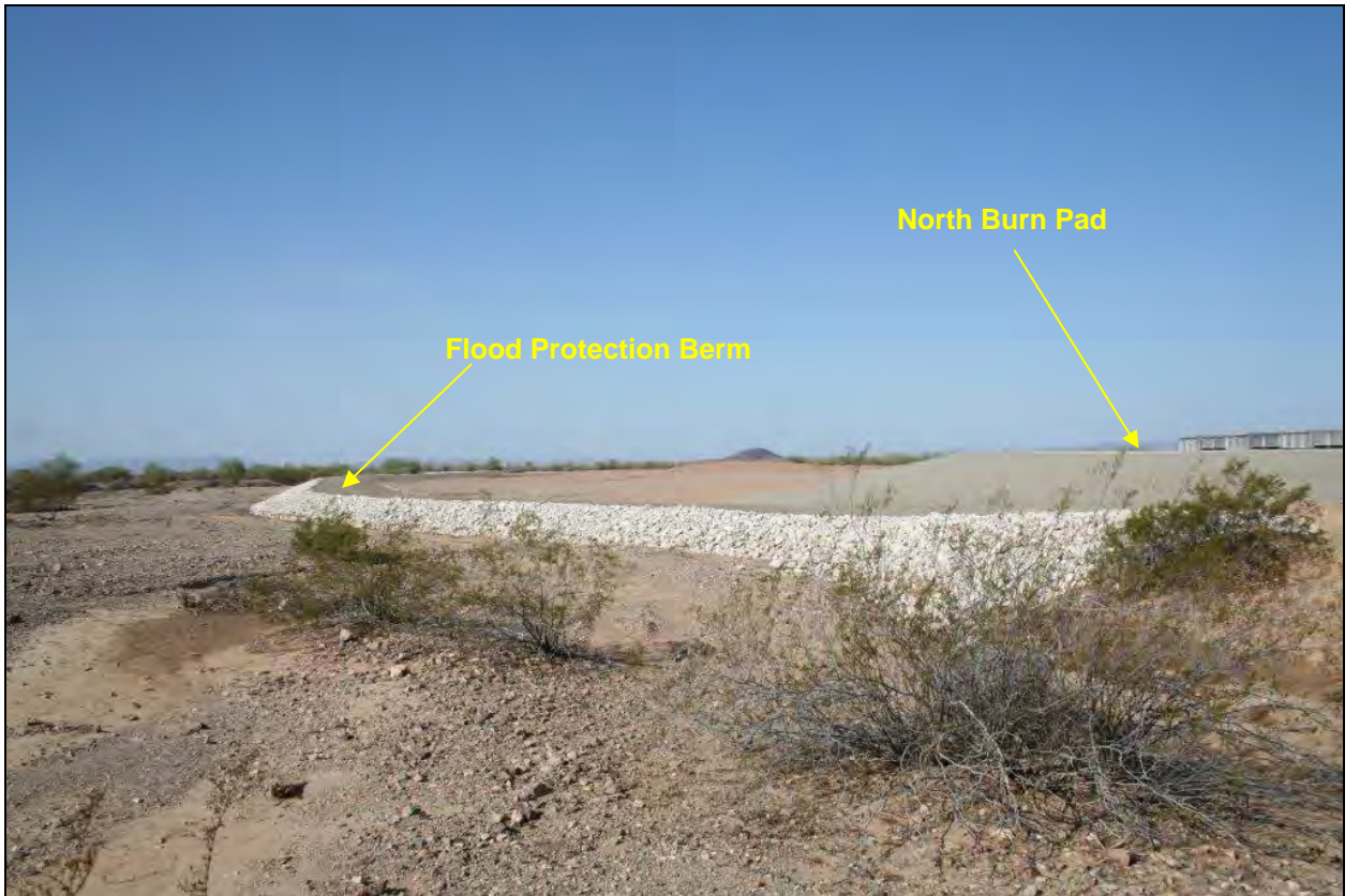
Photo 12 – Outside of Munitions Treatment Facility Flood Protection Berm Southwest of the North Burn Pad
