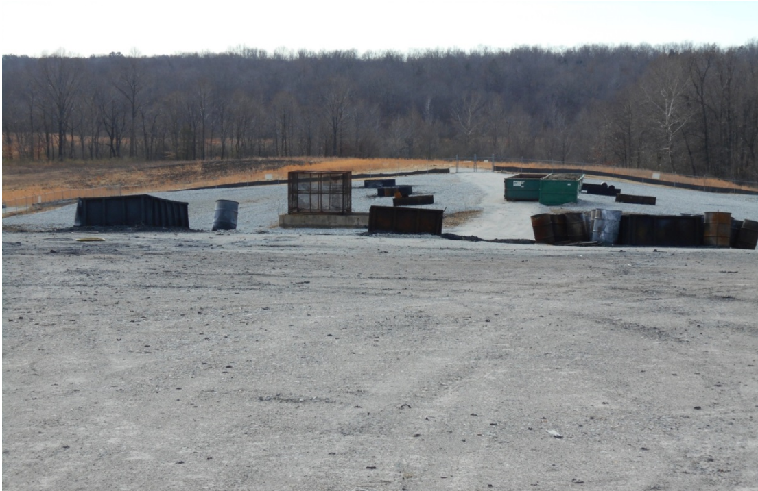
Photo 6: Picture taken looking south along the newly constructed road at the Hazardous Waste Open Burn Area south gate. (Photo taken 1-22-2014)
