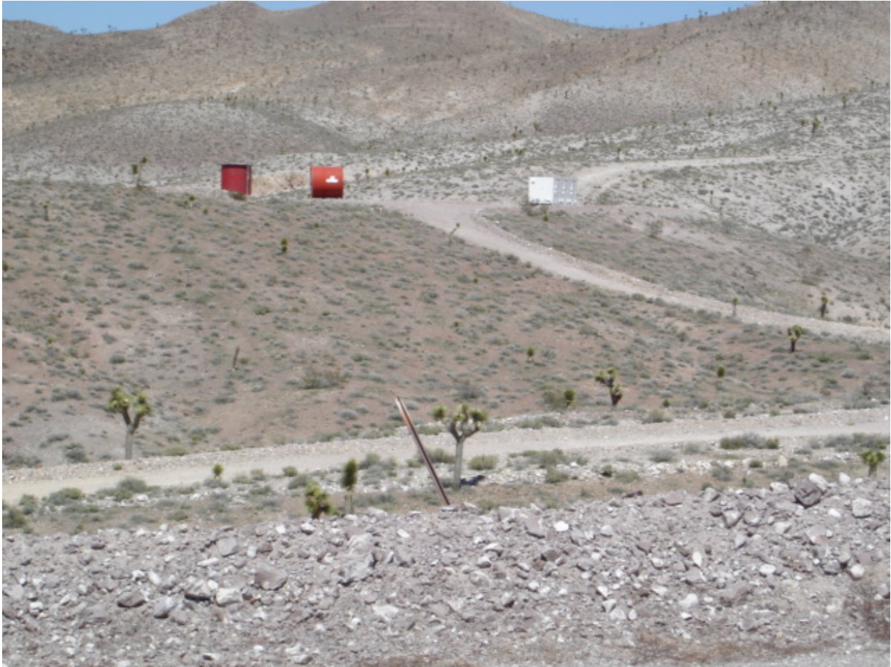
Figure 6. View of Storage Area
