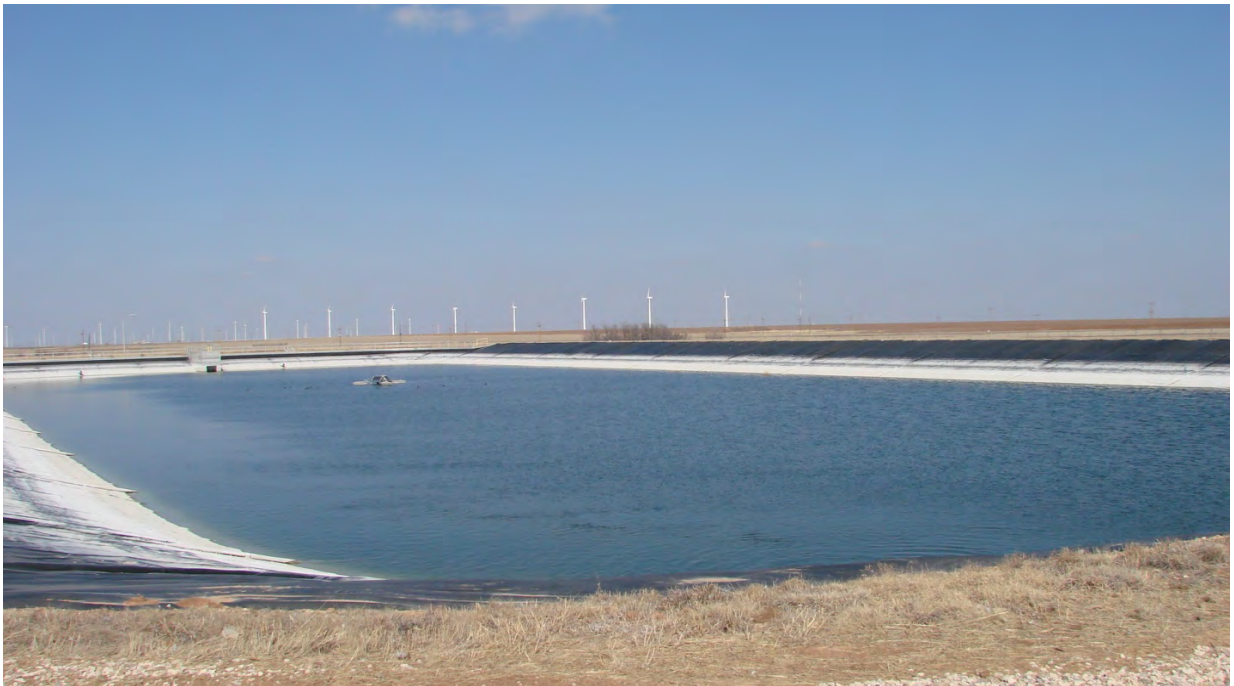
FIGURE 8.3 — East Wastewater Storage Lagoon
