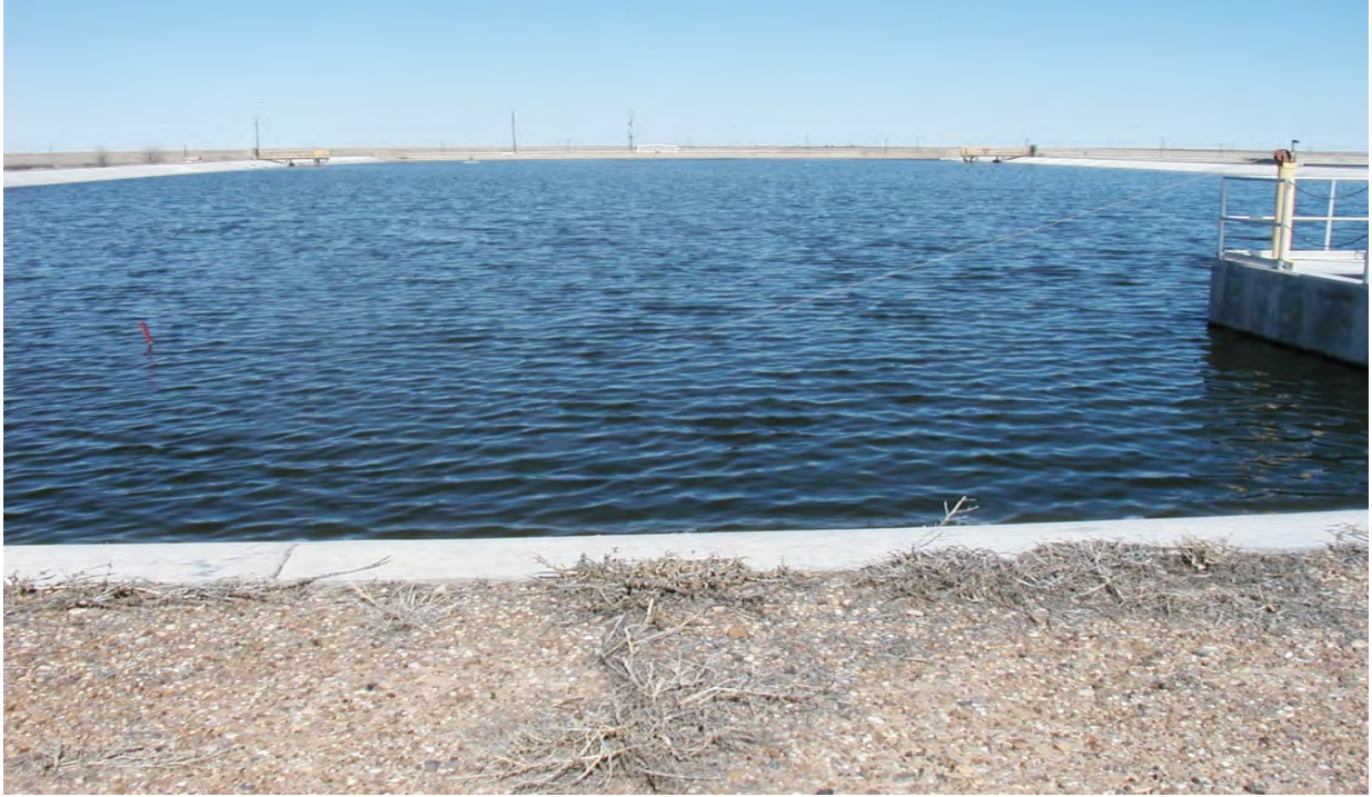
FIGURE 8.2 — Wastewater Treatment Facility, Facultative Lagoon
