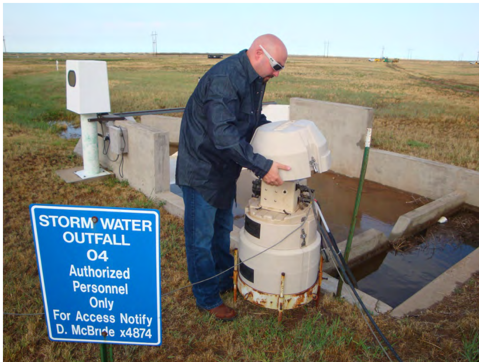
FIGURE 9.6 — Technician Checking Storm Water Outfall 04
