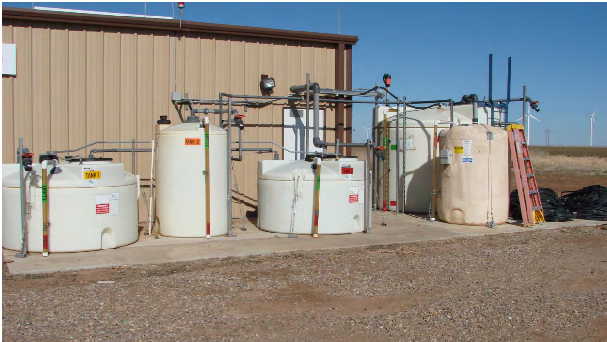
FIGURE 8.5 — Chemical Injection Tanks
