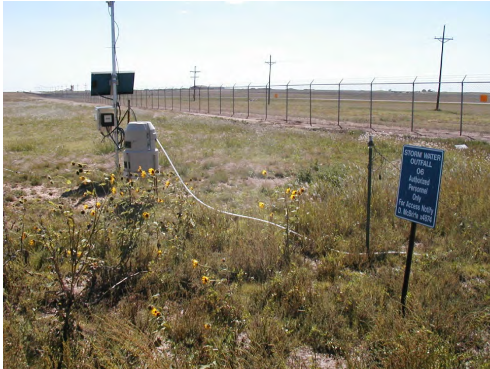
FIGURE 9.4 — Storm Water Outfall 06
