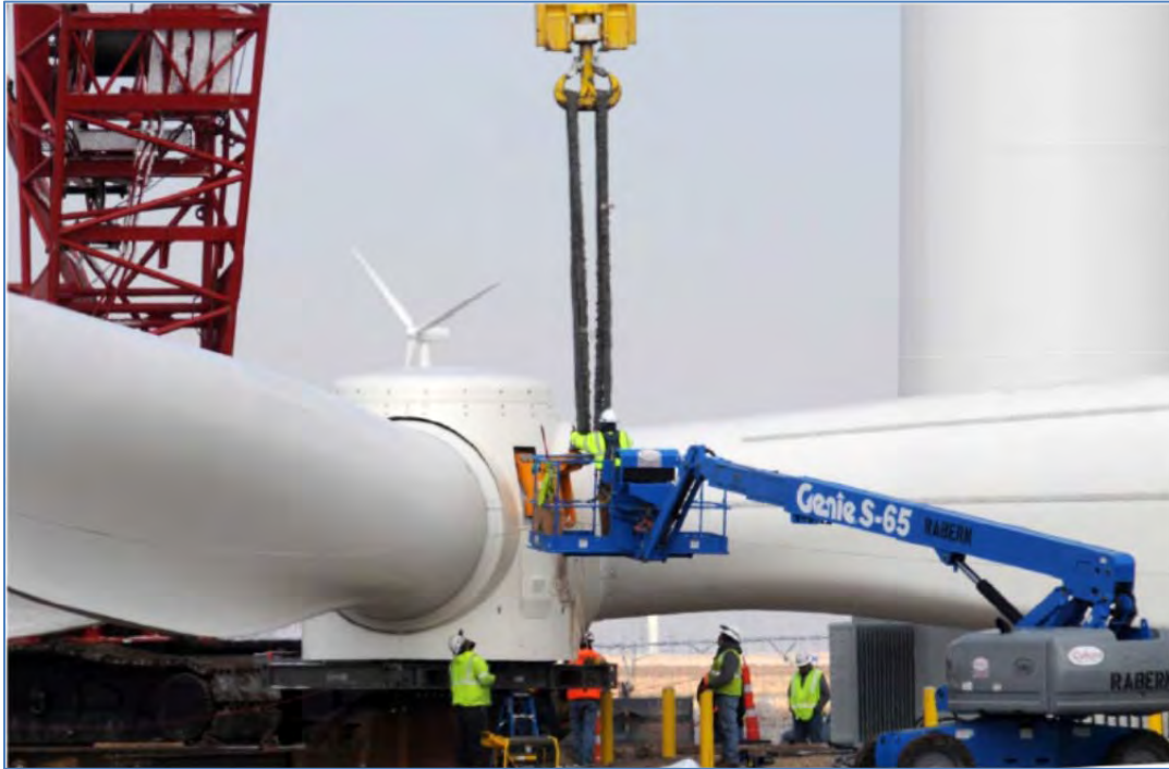
FIGURE 3.3 – Pantex Renewable Energy Project (Under Construction)
