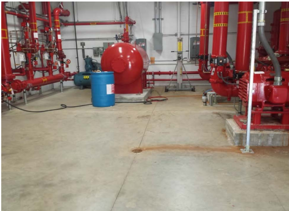
Photo 6: HEF storage (historically may have been AFFF storage) in the Mechanical Room of Hangar 406.
