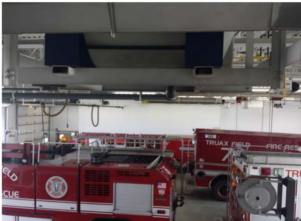
Photo 1: Overhead foam fill at Fire Station (Building 430).
