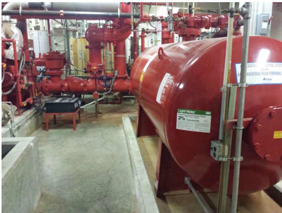
Photo 11: The AFFF fire suppression system at Hangar 208
