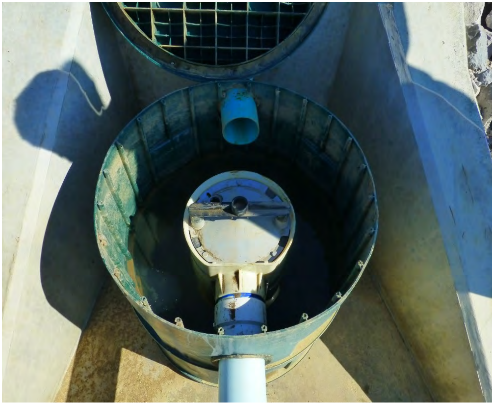
Photo 7: OB Unit - Sediment Catchment - Interior
