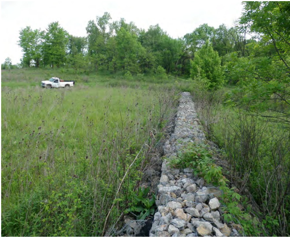
Photo 15: OD Unit - Looking North - Along Eastern Sediment Control (Rip-Rap)
