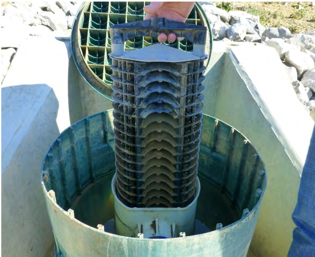
Photo 8: OB Unit - Sediment Catchment – Filter Basket
