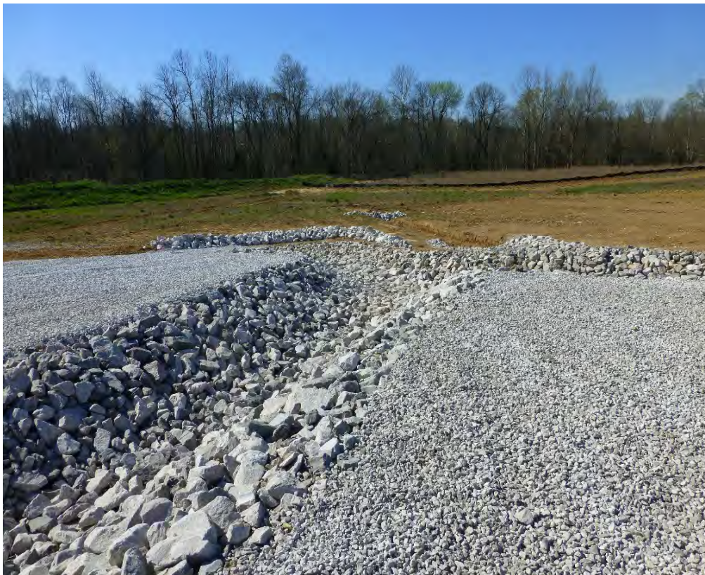
Photo 4: OB Unit – Looking South - Drainage Swale/Diversion
