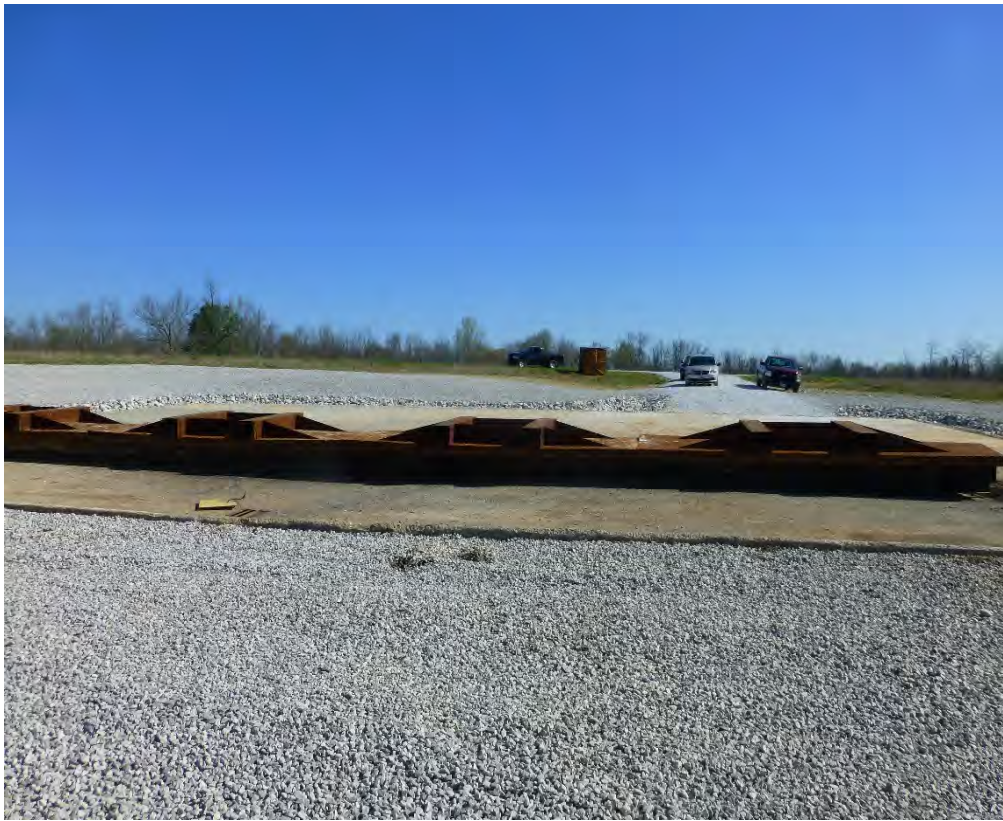
Photo 1: OB Unit – Looking North - Burn Pan with Lids and Crushed Stone Base Surrounding Pan
