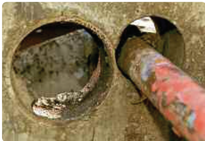
Catastrophic failure of primary containment bunding. © UK Health and Safety Executive
