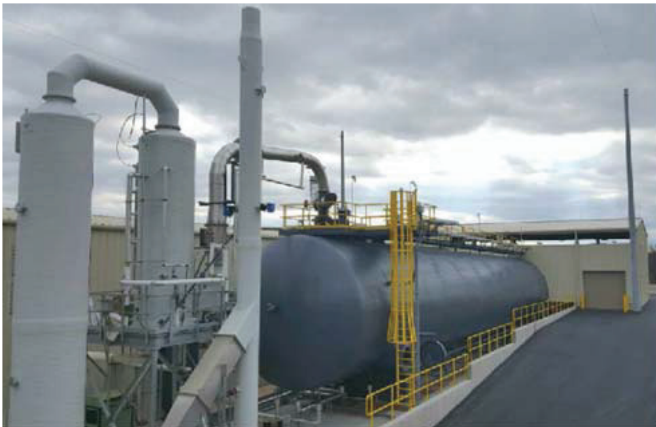
FIGURE 4.2 Ammonium Perchlorate Rocket Motor Destruction Facility thermal treatment chamber. SOURCE: R. Hayes, president, El Dorado Engineering, “El Dorado Engineering’s Technologies for the Demilitarization of Conventional Munitions,” presentation to the committee, October 24, 2017.
