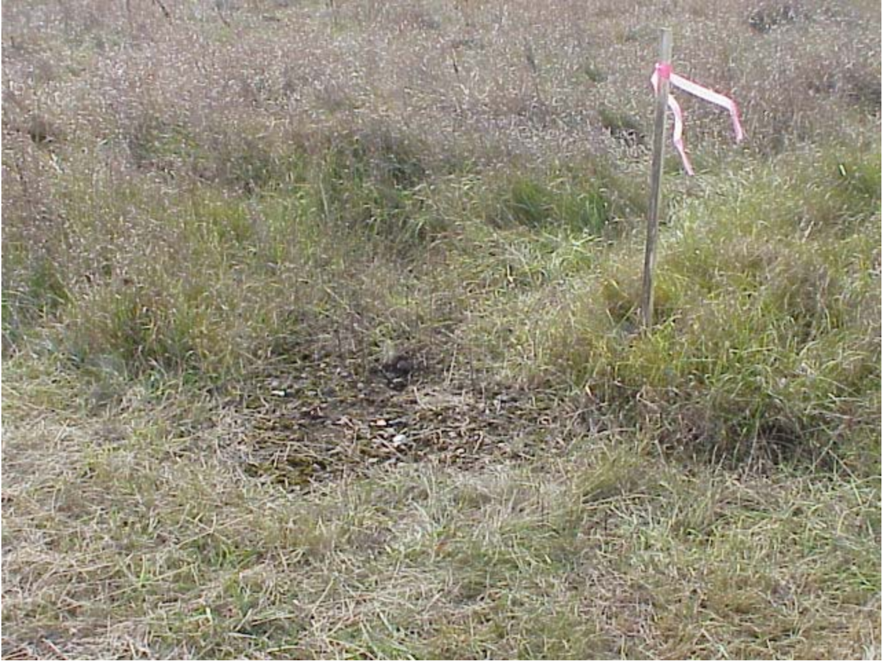
Distressed, circular, gravelly area just southwest of the rectangular concrete slab.
