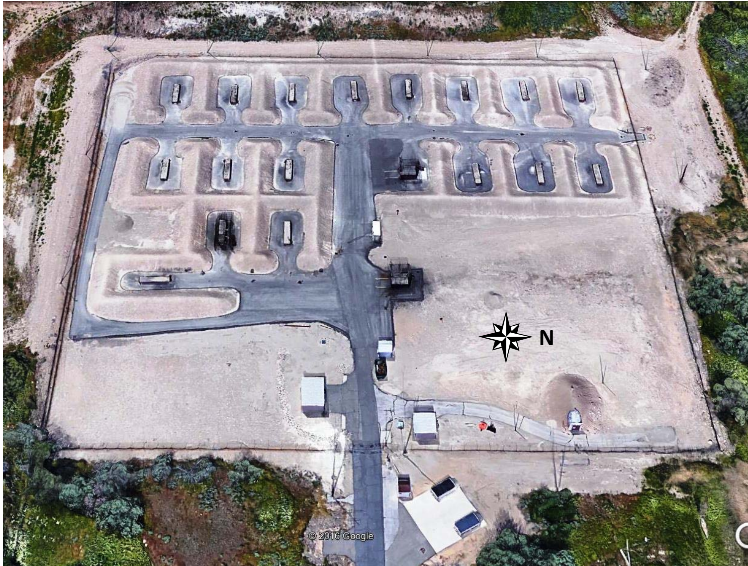
Figure 2-2.4 NIROP BURNING GROUNDS
