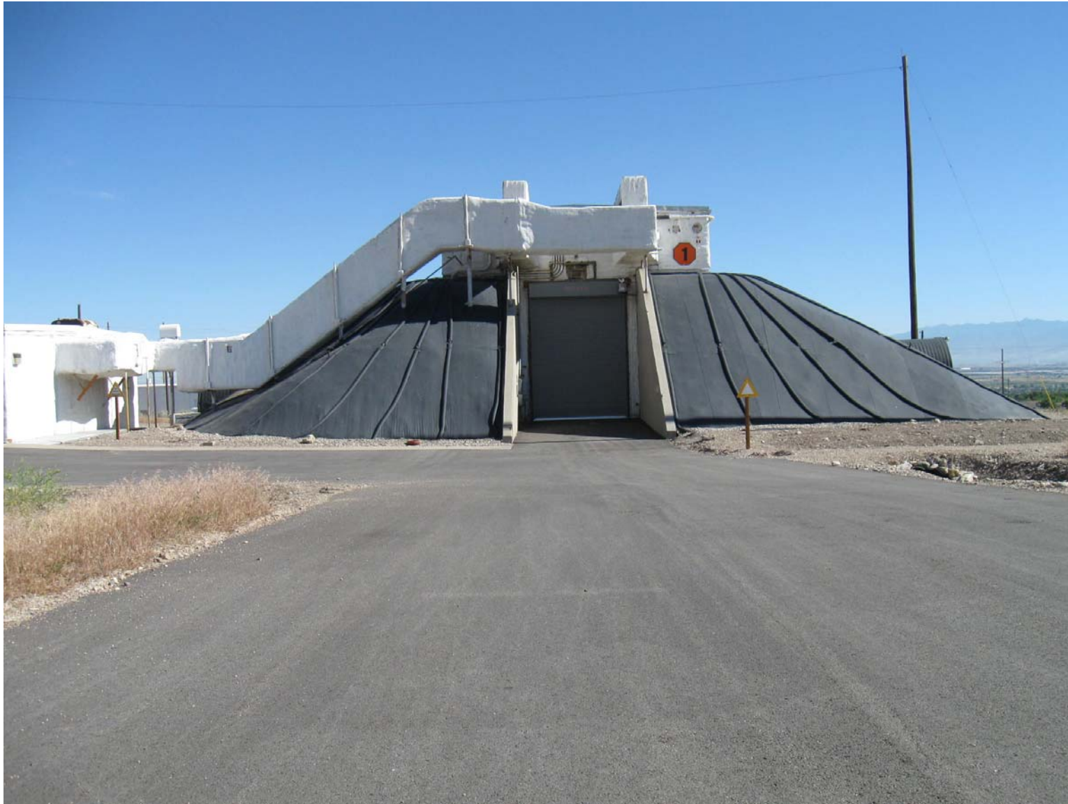
Figure 2-2.10 ES-3 Explosive Storage Building
