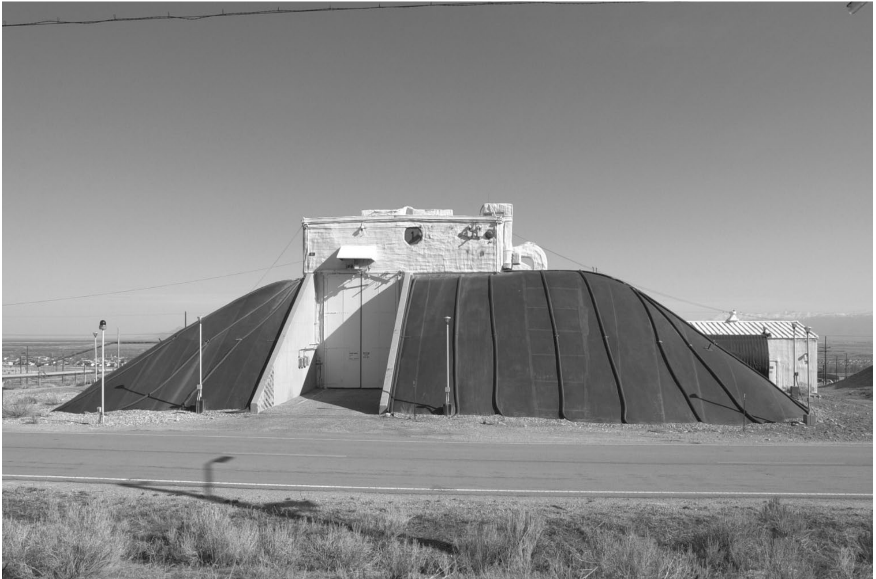
Figure 4-4.5 ES-2 Explosive Storage Building
