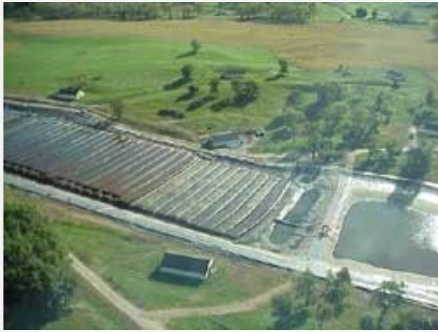
Aerial view of the geotextile tube laydown area and lagoon for dewatering contaminated sediments at Badger in 2001.
