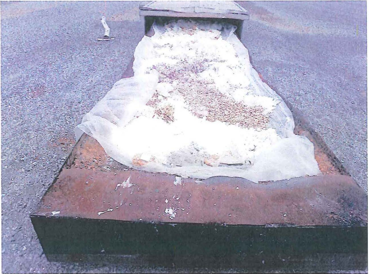
Picture 1: Holston Army Ammunition Plant – December 9, 2015 at 3:49 P.M. View of untreated waste in Pan 1 of the permitted Burning Ground unit. – Picture taken by Javier Garcia.
