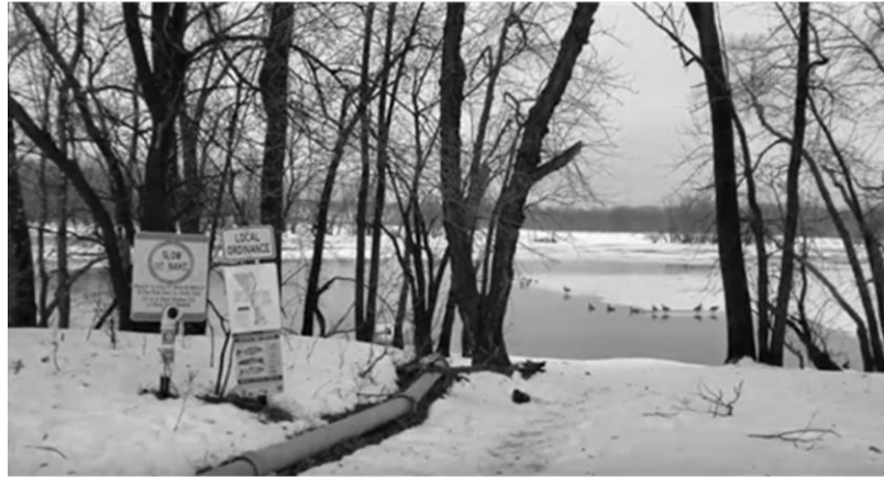
The City of La Crosse's Well #23 is located just east of the La Crosse Airport. Contaminated groundwater containing PFBS and other PFAS was piped and discharged directly into the Black River under a permit issued by DNR in June 2017. Outfall photographed in May 2019.
